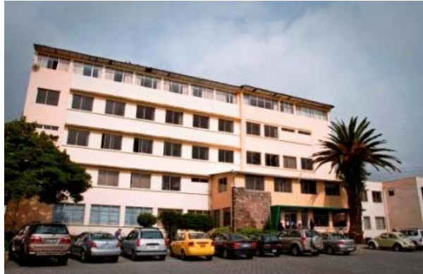
Fachada Hospital Pablo Arturo Suárez
