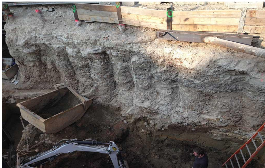
Figura N° 1: Columnas de Jet-Grouting. (Soperco, 2019)
