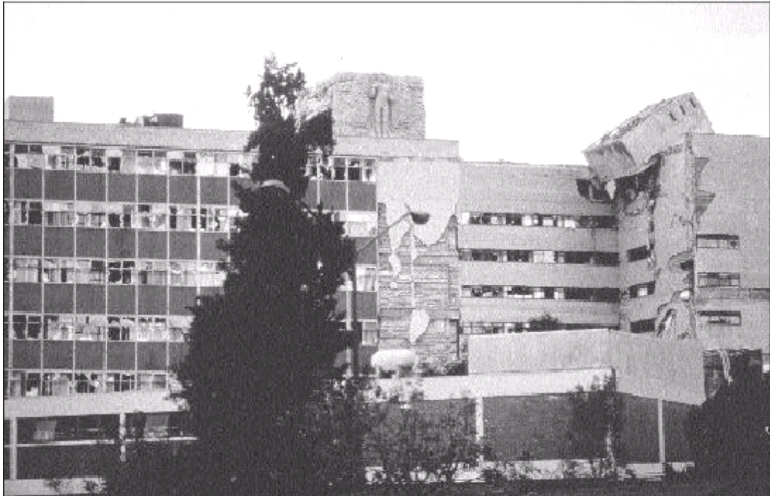
Photograph 8. Concentrations of mass, such as water tanks placed on the roof of a hospital, can cause severe damage in earthquakes.
