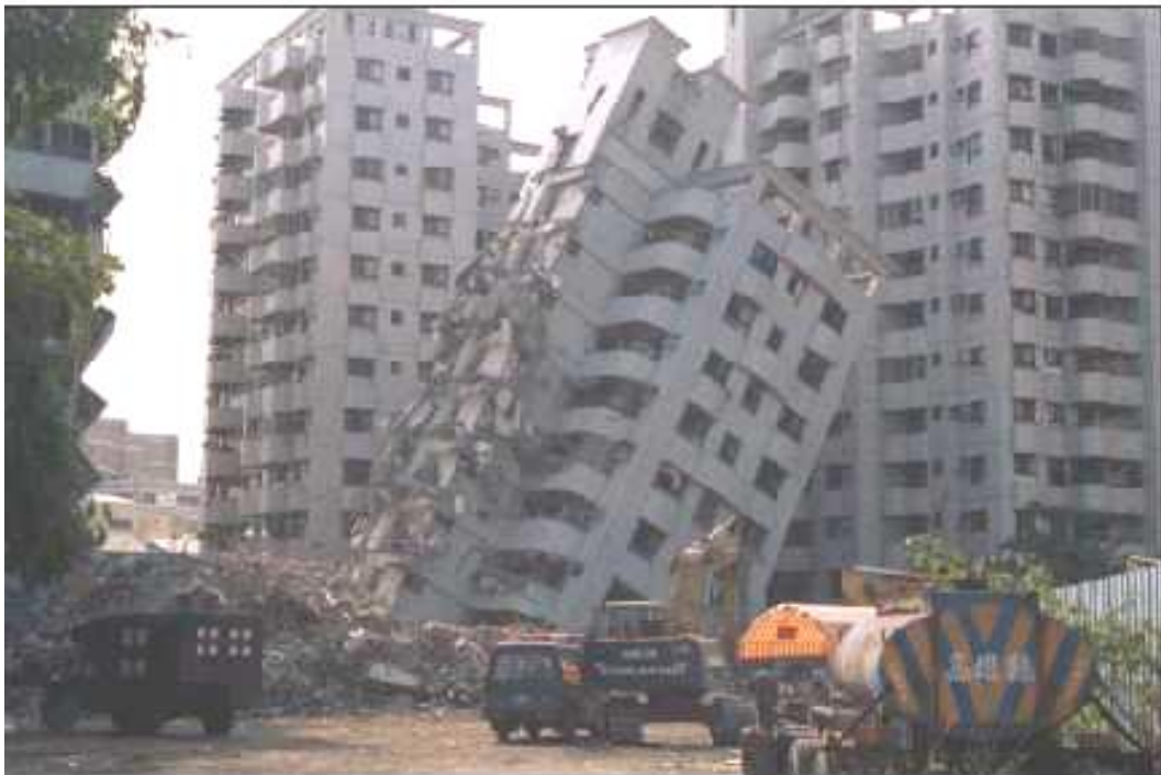
Figure 3. Failure of new construction.
