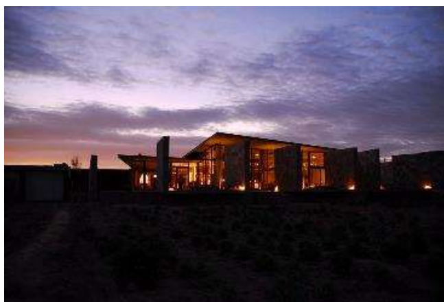
Figura 24: Vista nocturna Hotel Tierra Atacama
