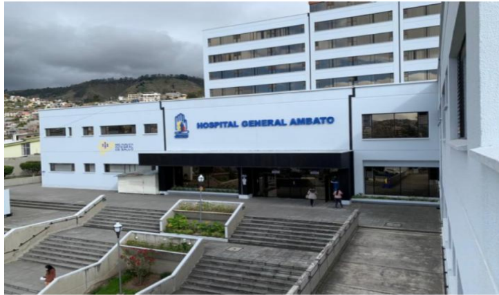
Figura 1. Hospital General Ambato
