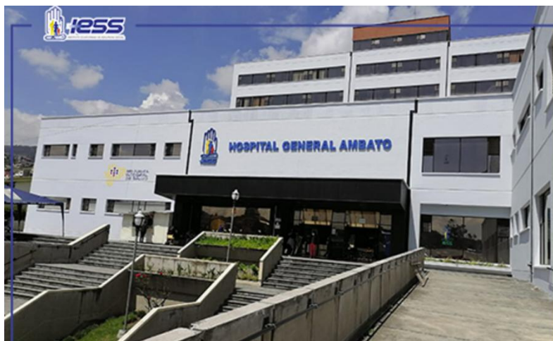
Figura 4. Fachada principal del Hospital General Ambato.
