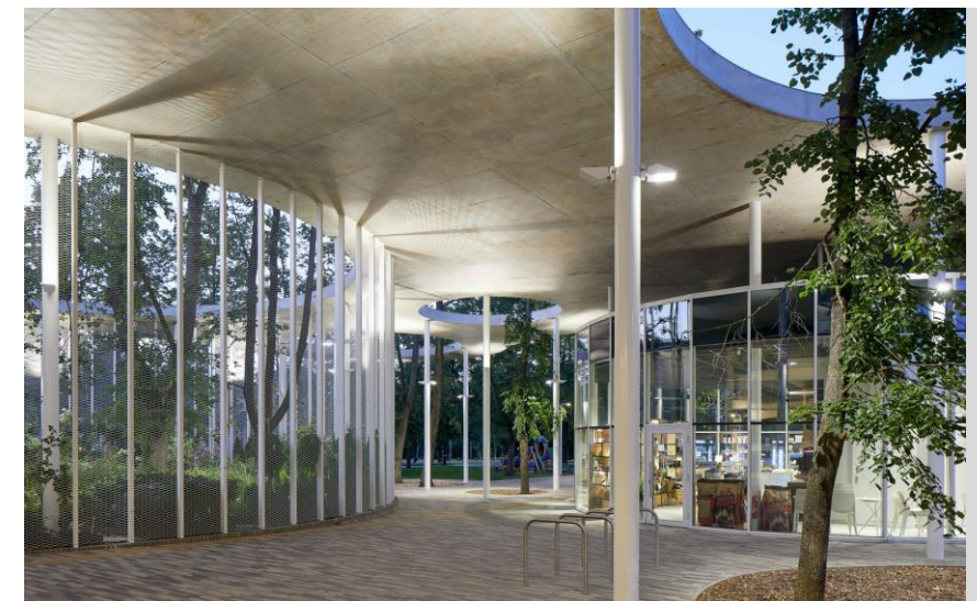
Figura 39: Vista interna de Vilkaividkid bus station
