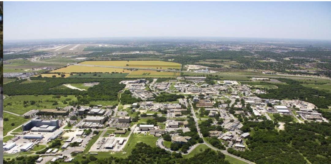
Pressure Tests Southwest Research Institute San Antonio, Texas
