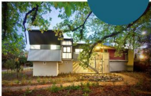
Perrera Stonnington | Architecture Matters
