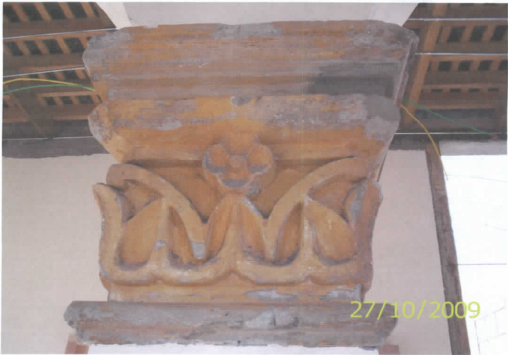
Detalle columna interior
