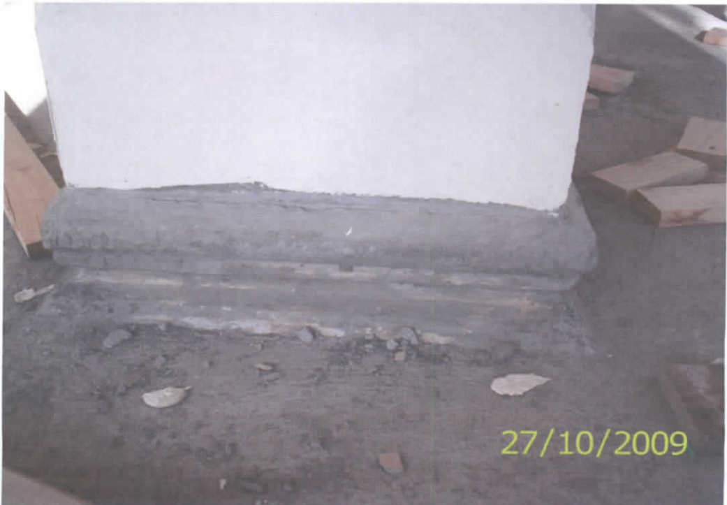
Detalle columna interior
