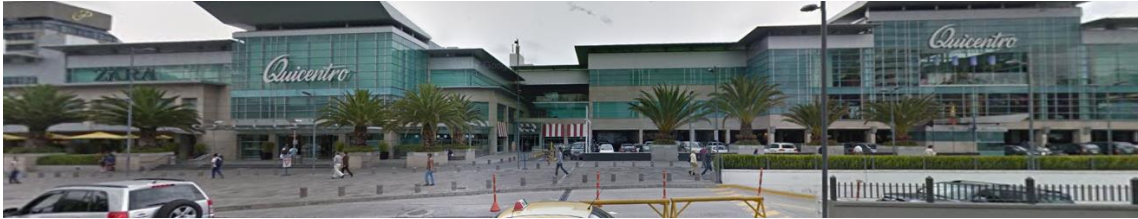
Figura 2: Centro Comercial Quicentro Shopping
