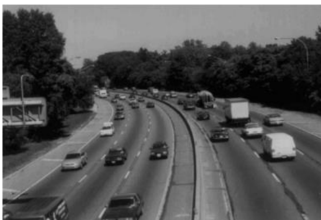
Figura 4. Nivel de servicio D. Tomado de: Highway Capacity Manual (HCM) (p. 131) por Transportation Research Board, 1994, The National Academies Press.
