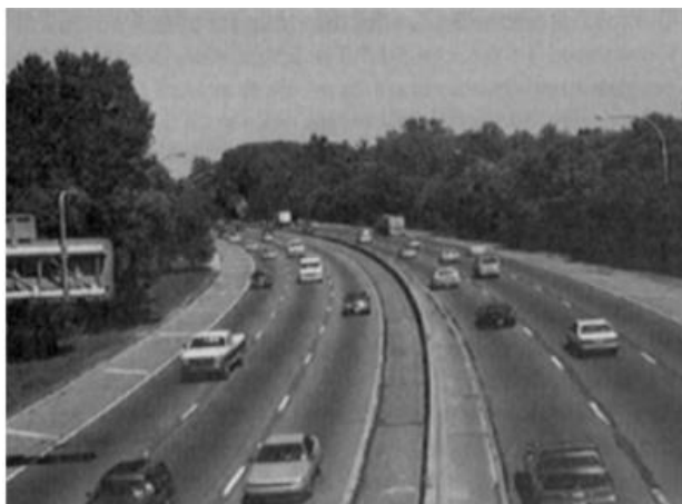
Figura 3. Nivel del Servicio C. Tomado de: Highway Capacity Manual (HCM) (p. 131) por Transportation Research Board, 1994, The National Academies Press.
