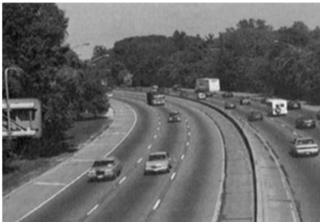
Figura 2. Nivel de Servicio B. Tomado de: Highway Capacity Manual (HCM) (p. 130) por Transportation Research Board, 1994, The National Academies Press.
