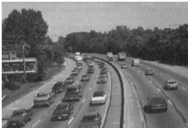
Figura 6. Nivel de Servicio F. Tomado de: Highway Capacity Manual (HCM) (p. 132) por Transportation Research Board, 1994, The National Academies Press.
