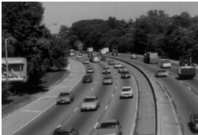
Figura 5. Nivel de Servicio E. Tomado de: Highway Capacity Manual (HCM) (p. 132) por Transportation Research Board, 1994, The National Academies Press.
