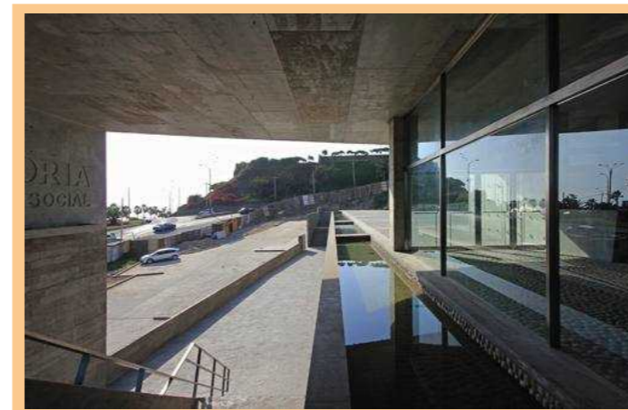
Fachada Frontal "LUM" Fuente: https://www.archdaily.com
